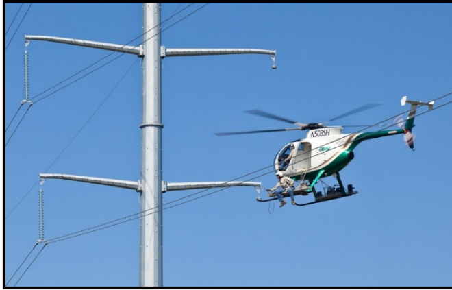
Helicopter at work installing spacers near Monticello, MN.
