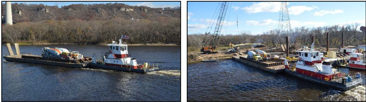
Figure 14: Barges were used to ferry equipment, materials, and labor to an island on the Mississippi River.
