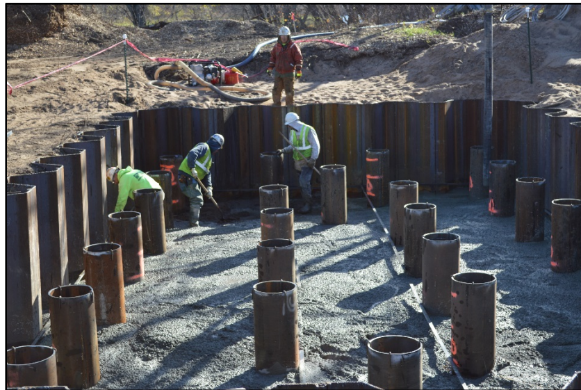
Figure 10: Construction crew pouring cement into a foundation
