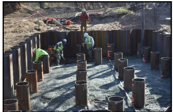
Construction crews pouring cement into a spread foundation as part of the Mississippi River crossing work
