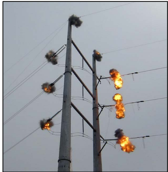
Figure 11: Implosive connector blast on a dead-end structure
